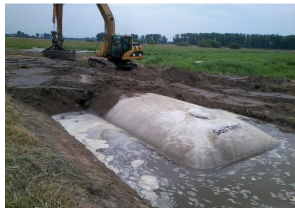
Photo 4 . Backfilling of excavation with filled SoilTain ® geotextile tube, Photo by WEMA
