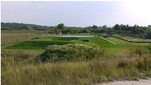
Fig. 5. Rostock research dike with filled polder 2, north view
